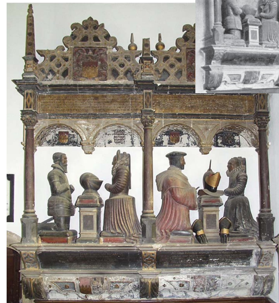
The earliest known photographic record of the monument c.1926, shows that the significant losses are historic. Later photographs confirm that the deterioration did not continue to a great extent after this date. The wall must have dried out, and the deterioration stabilised prior to this date.
